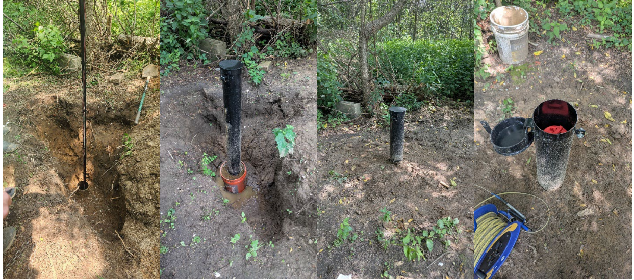
Figure 5. Photos documenting the Freedom_E well rehab and construction process.
